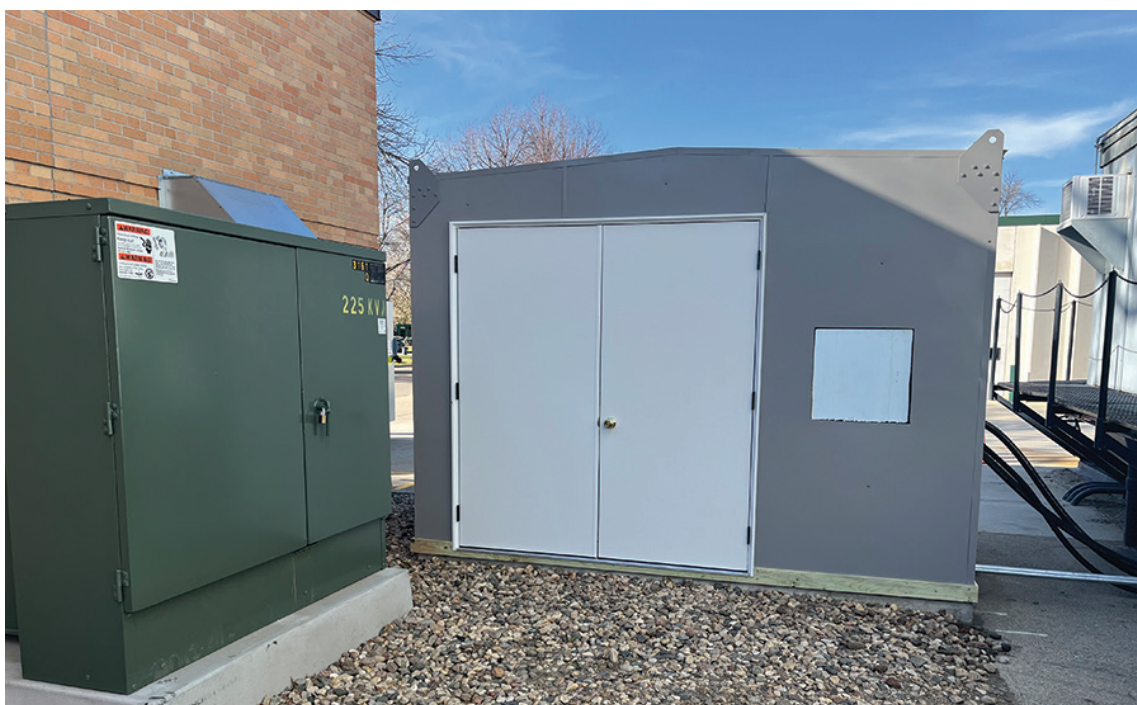
A view of the permanent shelter.
